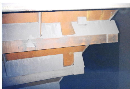
Fig. 8. Reinforcement of an industrial pyramidal bunker
