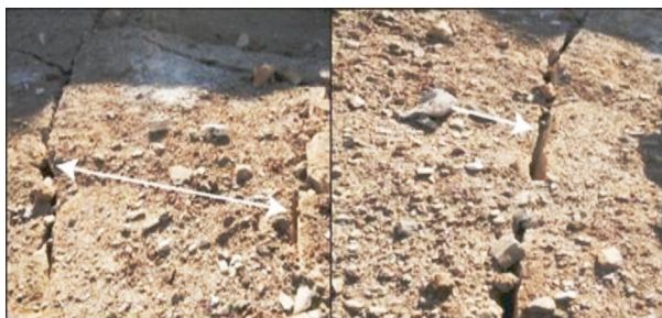
Fig. 8. Cracks created after blasting (Back effects)
